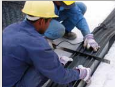
Melting of 2 elements with heating blade
