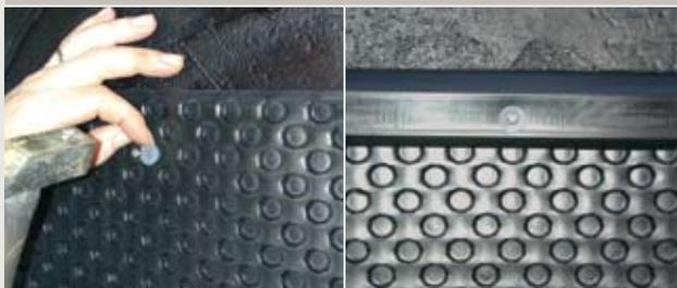
Fonda + membrane fixing by nails or Fonda wall plugs
