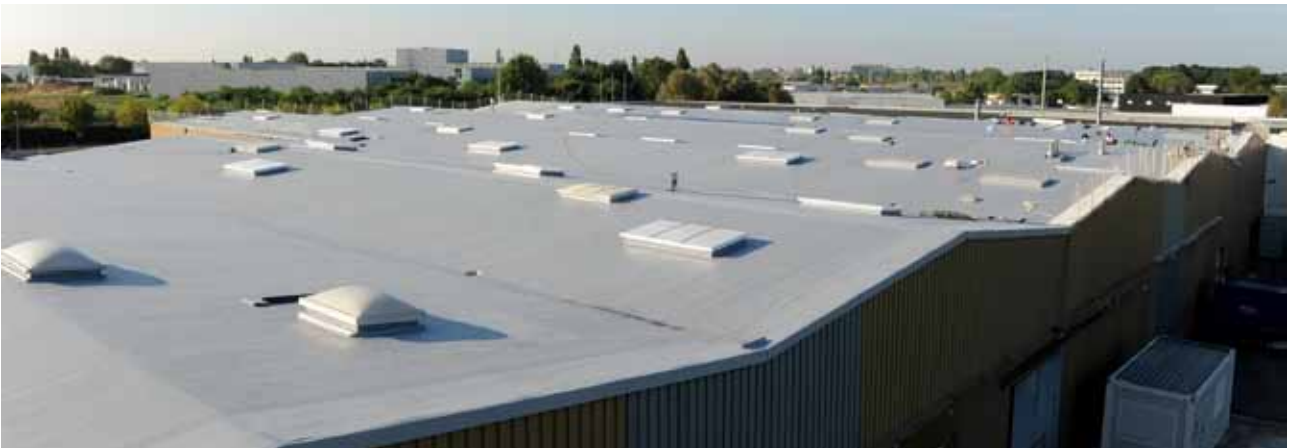
France , Rochefort, industrial building, 10 000 m 2
