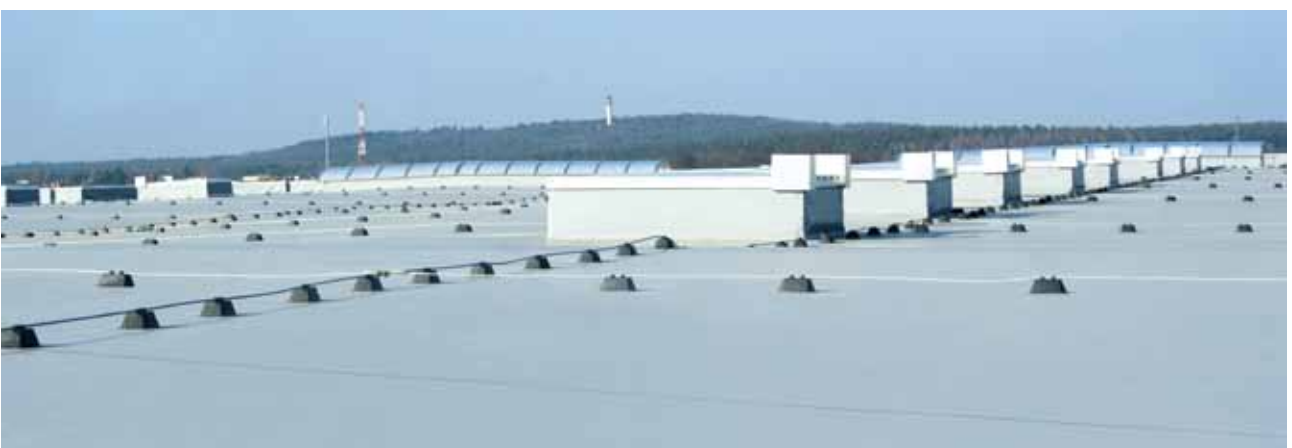
Poland , Komorniki, warehouse, 24 000 m 2
