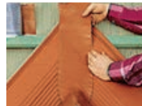
Push the product over the roof penetration and remove the release foil.
