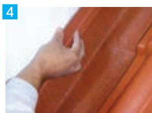
4 End with flashing and silicone bead.
