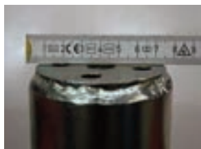
Measure the diameter of the roof penetration which has to be sealed.
