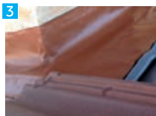
3 Detail of multipurpose waterproof strip joint.
