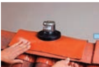
Mould Wakaflex® completely onto tiles without tension.
