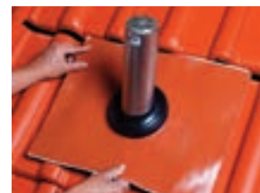
Push the product over the roof penetration.
