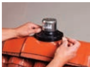
Install the cable tie below the border of the used diameter.
