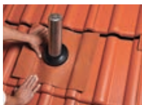
Mould Wakaflex® completely onto tiles without tension.
