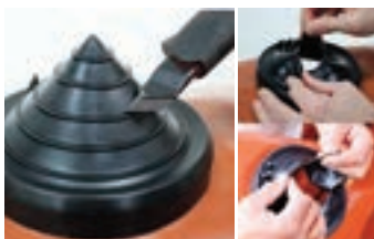
Cut the collar horizontally above the border line to the required size. The upper part of the collar can then be removed carefully by hand.
