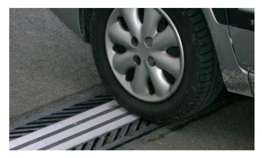
The flat joint seal is protected by PARADYL system: supporting plates of pultruded resin, supplemented by vulcanised elastomeric blocks with differentiated deformability, fitted onto the support plates plus installation of the pultruded resin covering bridge, fitted onto the elastomeric blocks.
