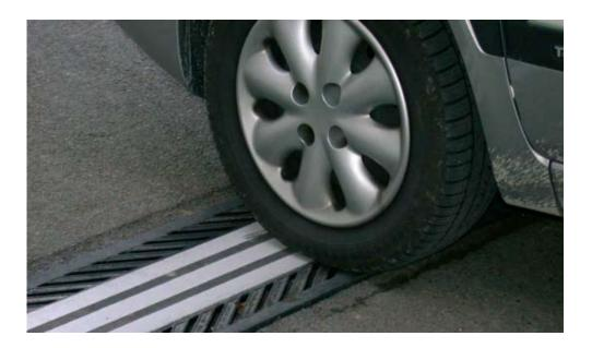
The flat joint seal is protected by PARADYL system: supporting plates of pultruded resin, supplemented by vulcanised elastomeric blocks with differentiated deformability, fitted onto the support plates plus installation of the pultruded resin covering bridge, fitted onto the elastomeric blocks.
